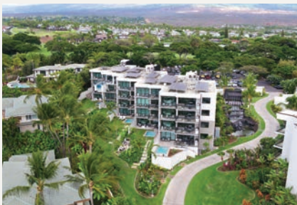
Andaz Maui, Wailea – Ilikai Villas Entrant: Nordic PCL Construction, Inc. and WCIT Architecture, Inc. Developer/Owner: Host Hotels & Resorts, Inc. Lead Design Firm: WCIT Architecture, Inc. General Contractor: Nordic PCL Construction Inc.
